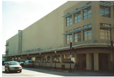
Savannah College of Art and Design's 85,000 square-foot Jen Library – one of the largest art school libraries in the country – occupies an entire city block downtown. It is housed in the former Levy and Maas Brothers Department store building.
